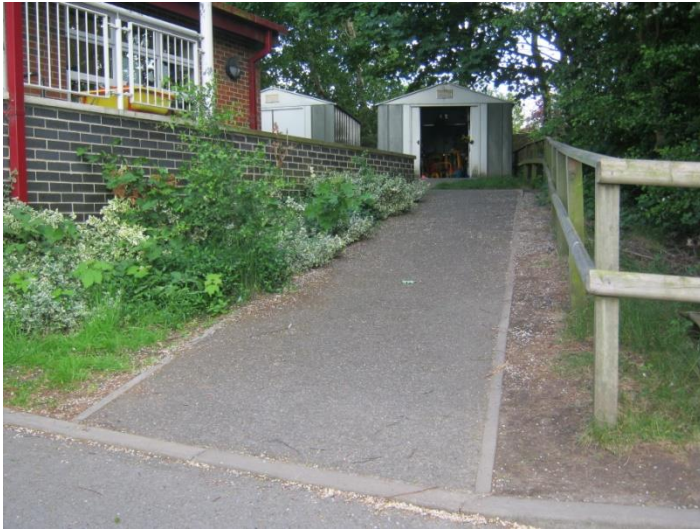
Access to RHS of top building
