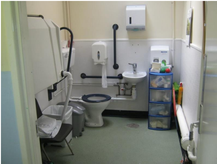
Accessible toilet – main building
